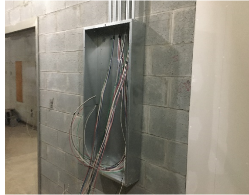
Electric Panels Wiring
