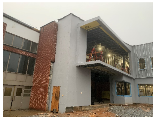
New Addition Air & Weather Barrier
