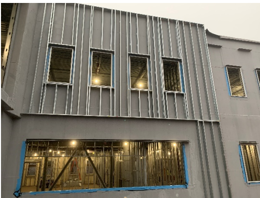
New Addition Precast Stone Framing
